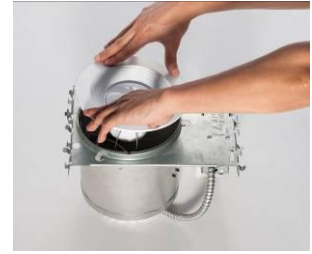
Step2: Insert male connector into female one.
