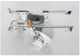
Step 2: Insert the male connector into the female one.
